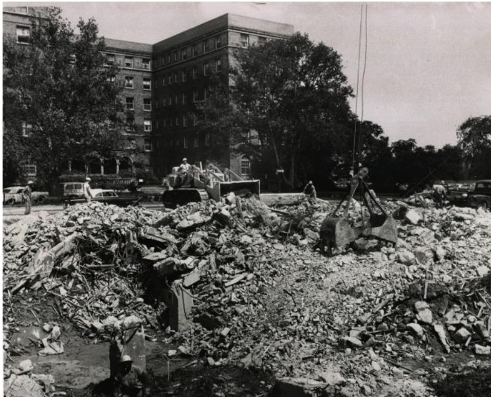
Site of demolished Gotham Hotel in 1963.
